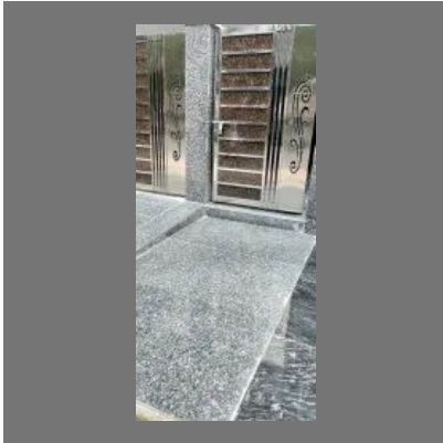
Ss Main Gate
